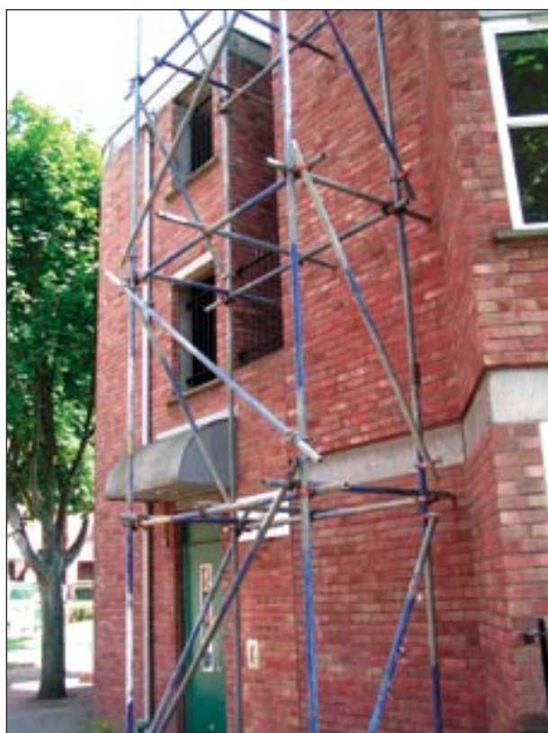
▲ Scaffolding at 300 Ladbroke Grove
